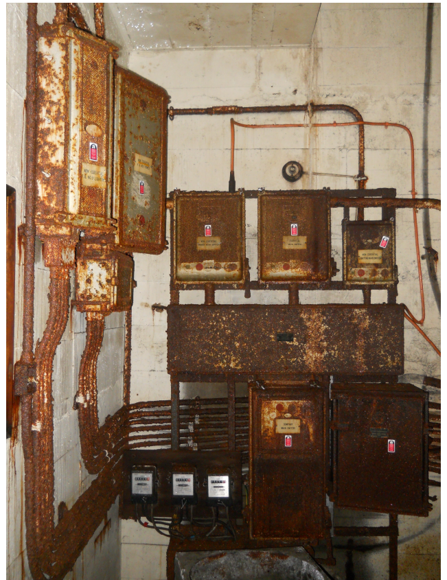
Main fuses (bottom of emergency stairs) 23 June 2016 (Photo: Bill Ridgeway) (1402)
