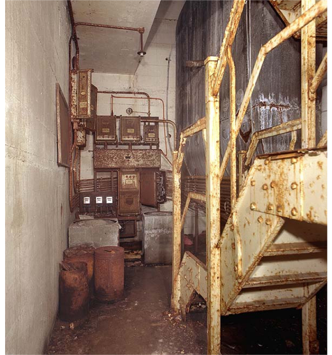
Main fuses (bottom of emergency stairs) c 2001 (Photo Nick Catford) (266)
